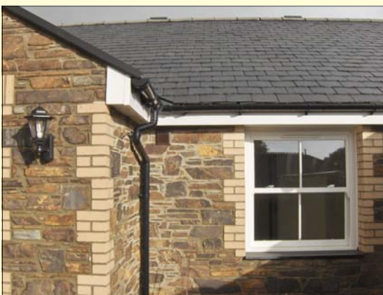
Low maintenance exterior
